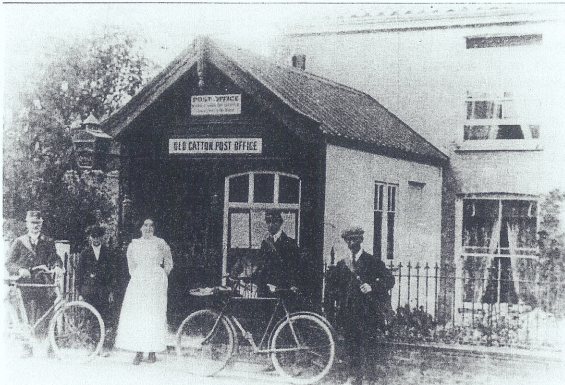
The Post Office about 1914-18 (since demolished) House at the back is now No 125 Constitution Hill
