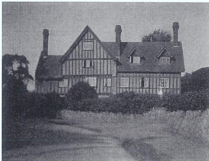
Manor House, Church Street
